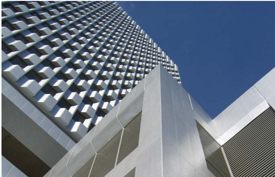
Steel and concrete substrates
